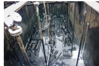
Old diffuser system prior to reconstruction
